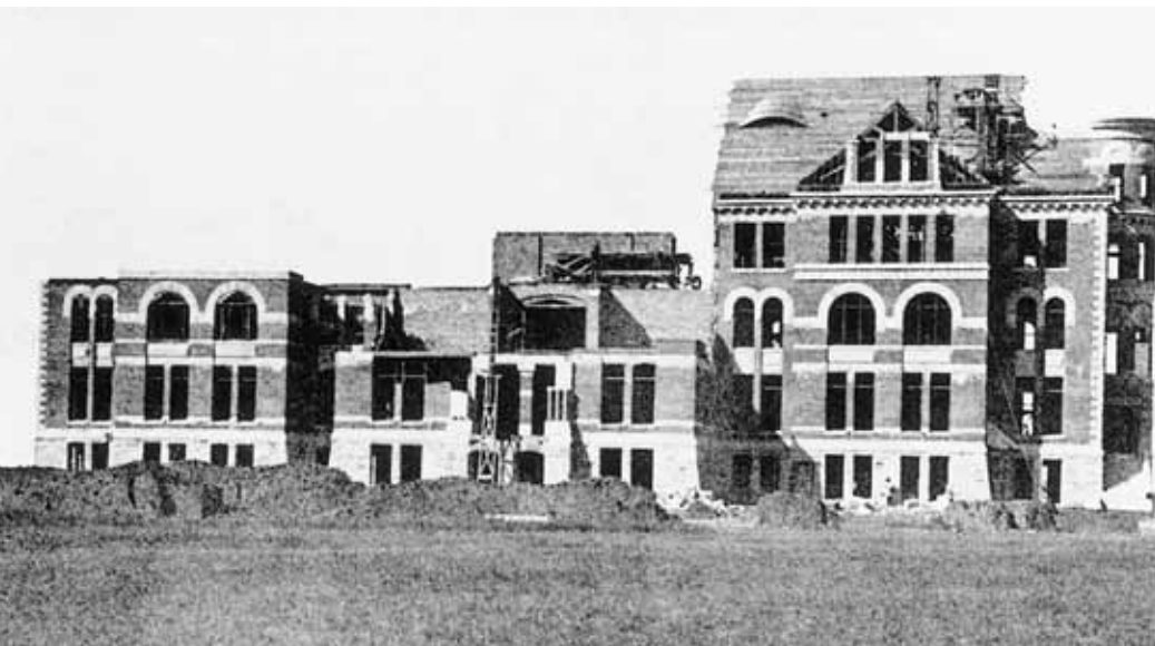
The Davis Administration Building (then Garfield University) under construction in 1886.
