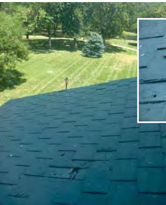
The July 8 hail storm severely damaged the Davis Administration Building’s slate roof. This photo was taken from the fourth-floor northeast window, overlooking the lawn south of the Riney Fine Arts Center. The Vermont Black slate ranges in size up to 18 inches and is approximately one-quarter inch thick.
